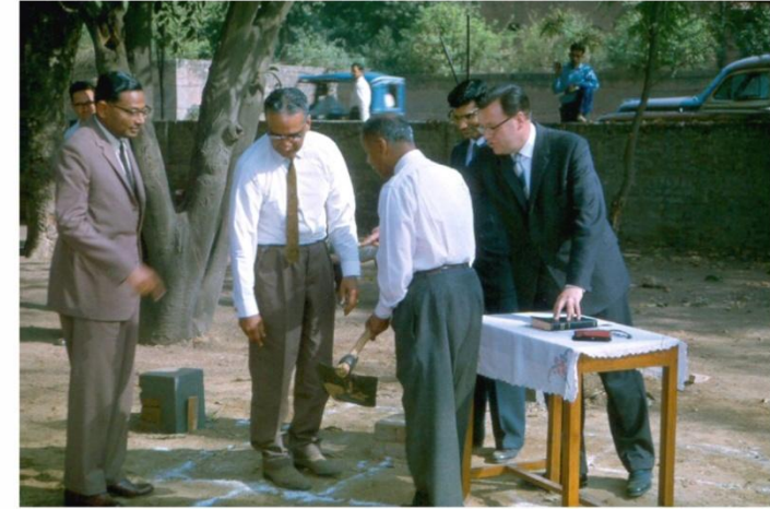
Cutting the first sod
